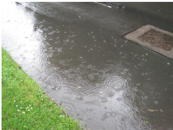
Combinations of ineffective drain clearance, ineffective capacity showing surface water continuing in roadway. With only a 6" pipe the system is never able to cope with water under moderate/heavy rain conditions. This has given rise to sewerage problems on several occasions further along Blunham Road.
