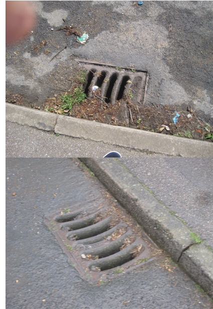
Typical of many other drains along this road choked with grass, leaves and soil
