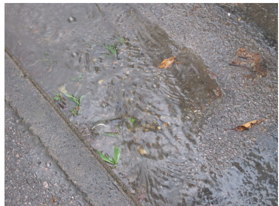
Combinations of ineffective drain clearance, ineffective capacity showing surface water continuing in roadway. With only a 6" pipe the system is never able to cope with water under moderate/heavy rain conditions. This has given rise to sewerage problems on several occasions further along Blunham Road.
